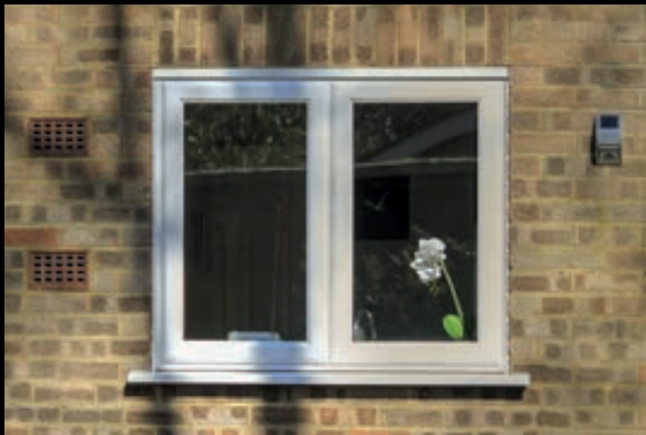
The floating central mullion allows the windows to benefit from the maximum opening without obstruction.
