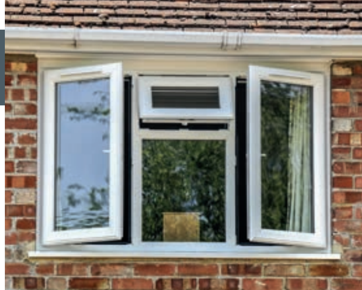
Trickle Vents installed through the window sashes
